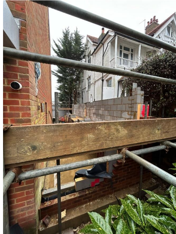
Progress of construction
