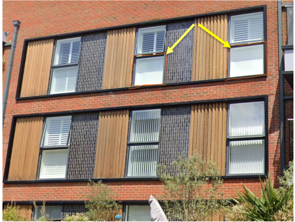
Window elements with grey aluminium frames highlighted
