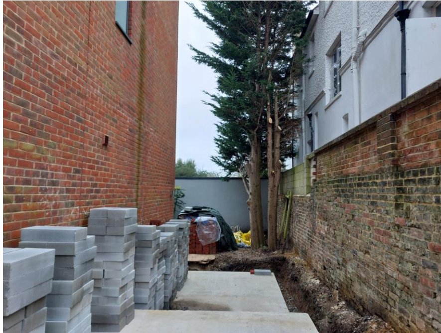
Progress of construction
